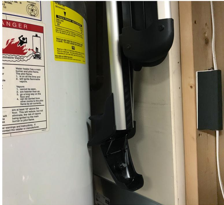
Fig. 11. A possible implementation of a temperature monitor deployed on a stud (location E)
